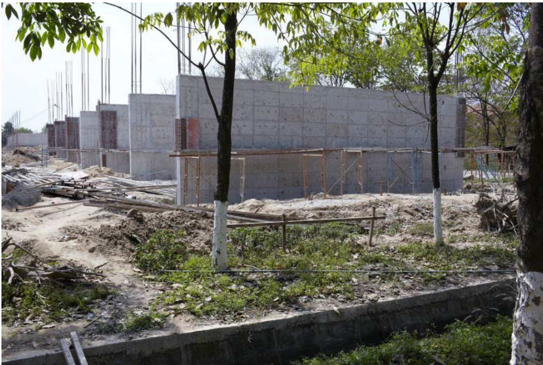
Figure 4 Composting building under construction in early 2012. (Source: Jussi Kukkula, Ferroplan)
