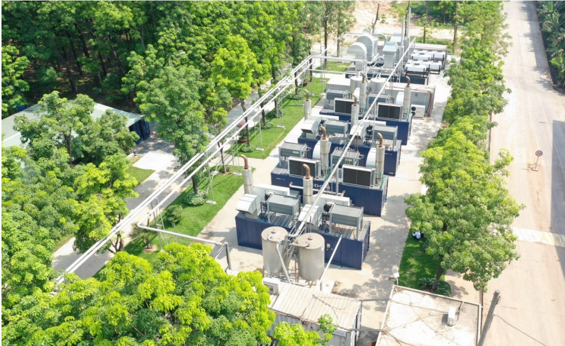
Figure 12 The CHP units and related infrastructure in 2021. In the front are the filters installed during the CCS project. The blue containers are the CCS project installed capacity of 1 600 kW and the black containers in the back the additional 720kW implemented in the EEP financed project. (Source: Hoai Le, evaluation team)
