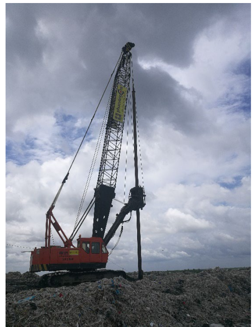
Figure 10 Drilling the gas collection wells. (Source: Doranova Oy)
