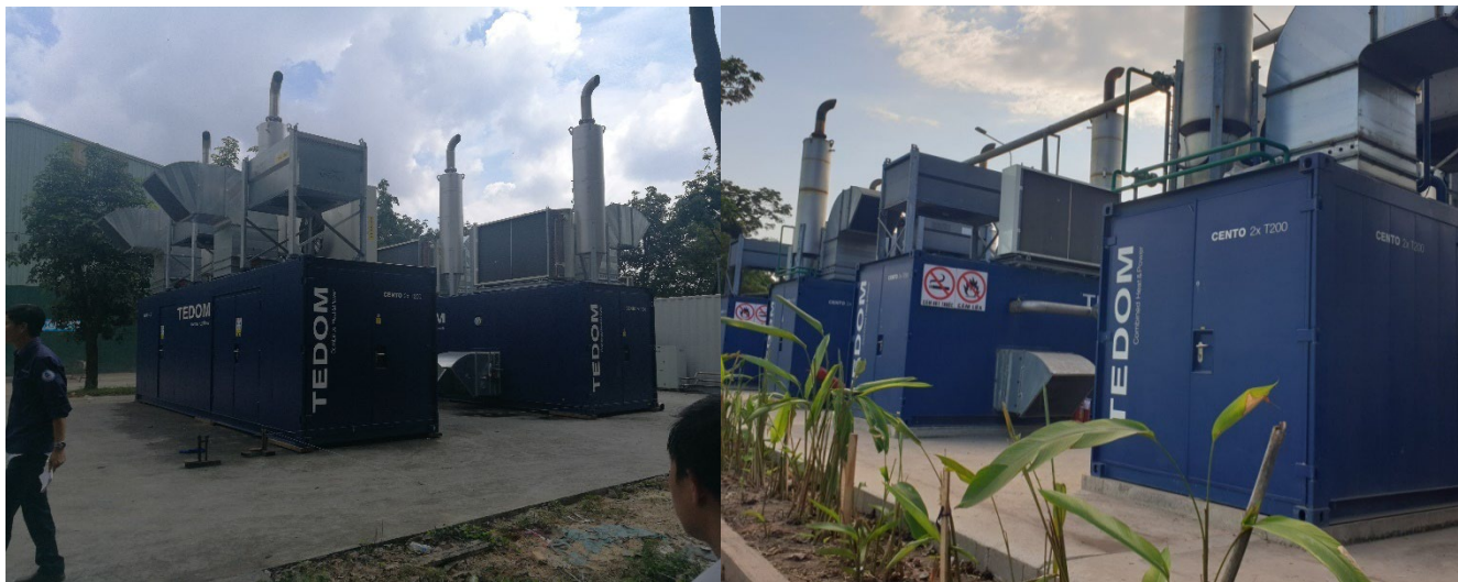
Figure 20 CHP units in 2018 and in 2021 (Sources: Doranova Oy and Hoai Le, evaluation team)
